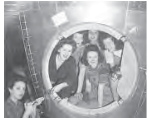
This 1944 photo shows female workers with an airline fuselage at the Kenworth plant, South Lake Union. Do you know anyone who has a story to tell about working at one of the many industrial plants around Lake Union?
